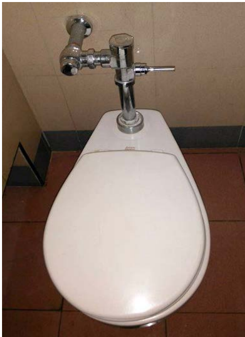
MANUALLY ACTIVATED FOM VALVE TOILET
