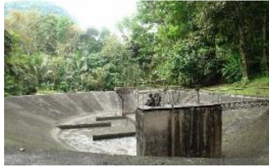
FIGURE 1 OLD RESERVOIR / SAND AND GRIT REMOVAL BASIN
