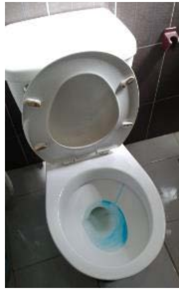
TOILET WITH LEAK AFTER DYE TEST
