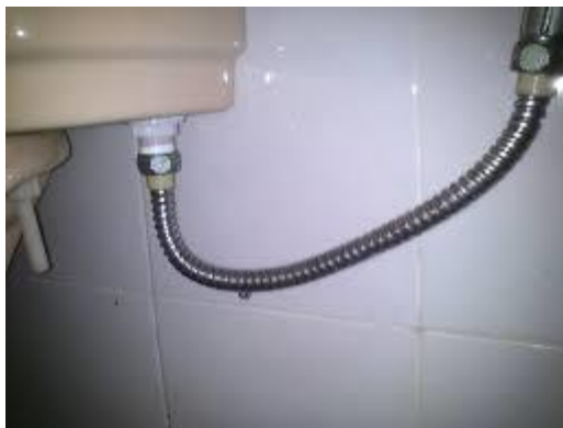
WATER LEAK AT THE CONNECTION HOSE
